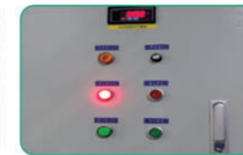
Variable frequency transformation of air conditioning pump transformation
